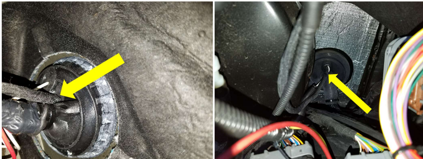
Figures 5a & 6b - Wire Bundle under Dash and in Engine Bay
