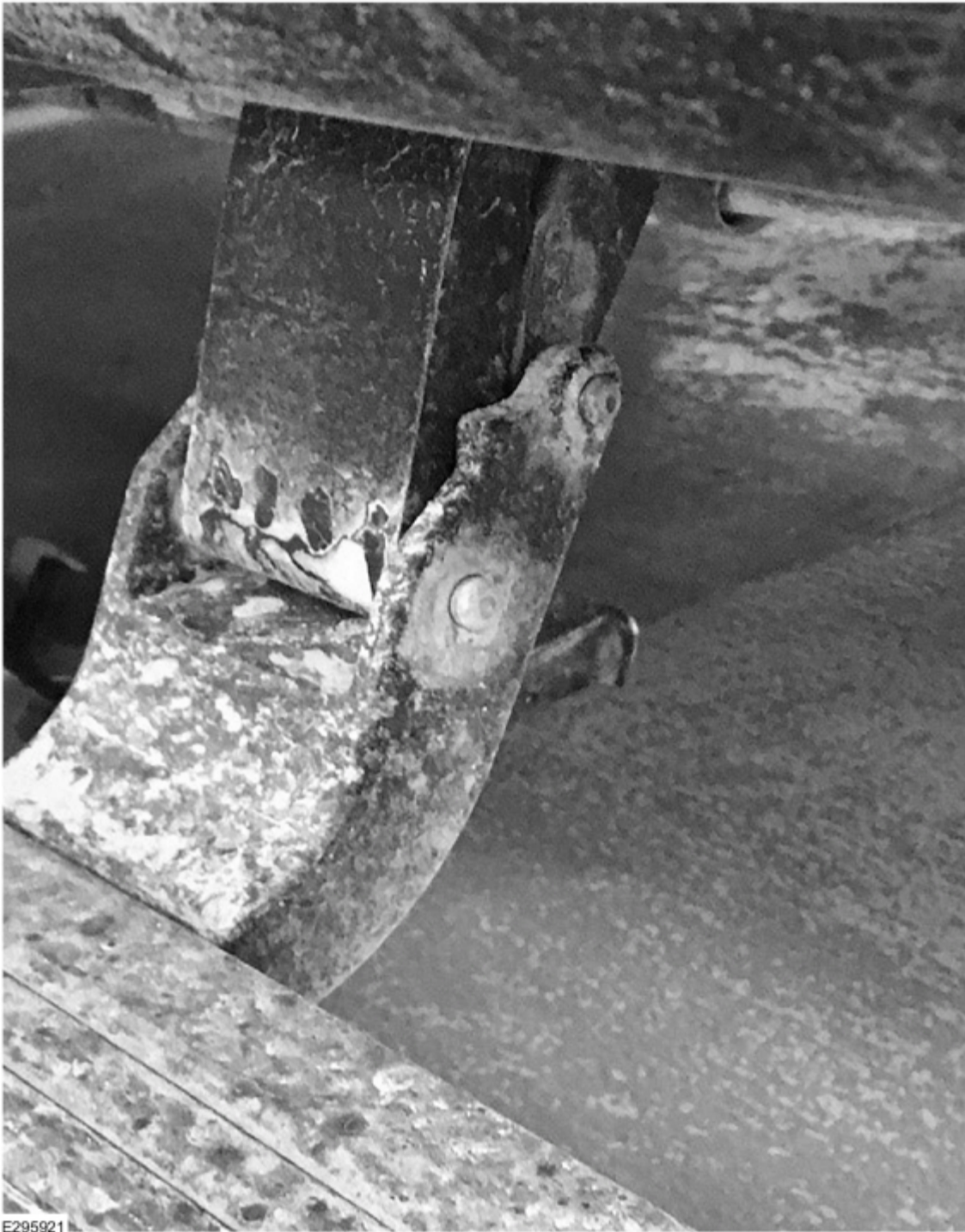
Clean running board after pressure washing (Figure 2)
